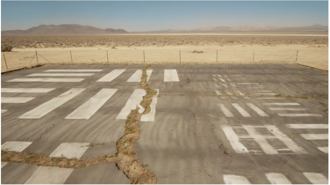
Figure 4. Still from Hito Steyerl, How Not to Be Seen: A Fucking Didactic Educational .MOV File , 2013. Single-screen video. This is a resolution target paved onto ground of the Californian desert. It cracks demonstrate its disuse, as this type of image resolution calibration is no longer in use.
